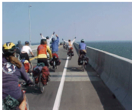
Crossing the Confederation Bridge to PEI Photo submitted by Rob McLean
